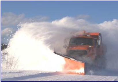
Under contract, Alcona County Road Commission maintains the state trunkline, including snow removal.
