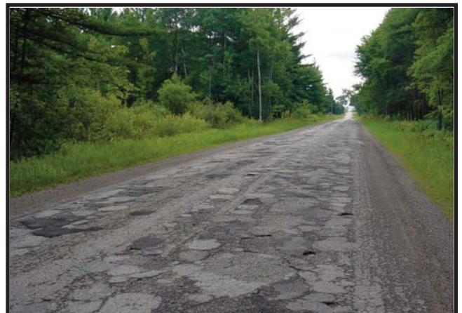
This Wexford County Road was returned to gravel in 2008 due to the lack of funds for maintenance.
